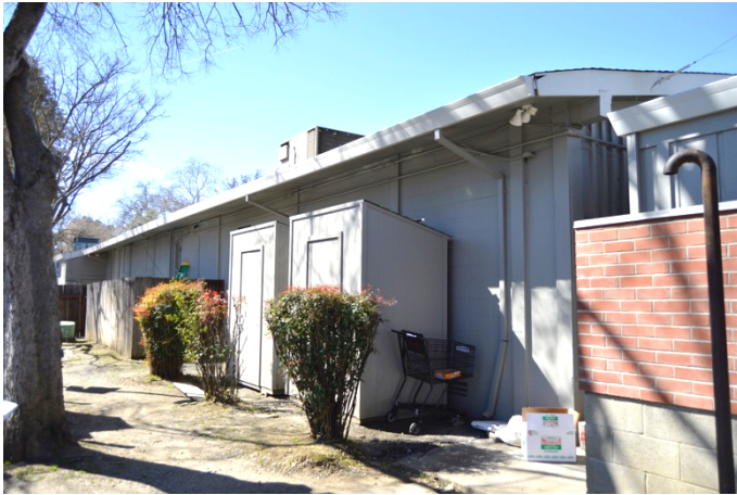
Figure 3. Rear of building is not fenestrated.
